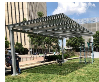
Finishing touches for the pergola at Chapman Green
