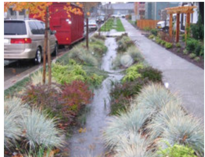
Example of Bioswale which catches rainwater from the street. Source: https://www.centralcoastlidi.org/landscape.php
