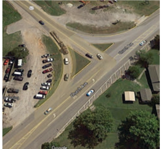
Intersection of Church Avenue and Highway 62 where the proposed roundabout is located. Source: Google Earth
