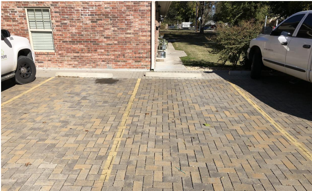
Parking lot with pervious pavers
