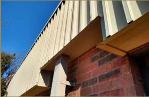
reference photo of 6"x4" gutter and metal roof flashing
