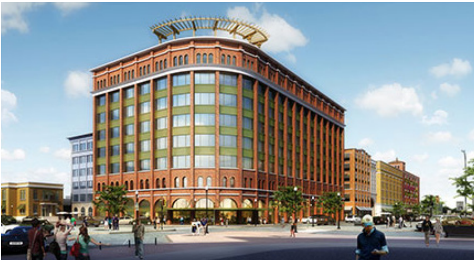
Above and Right: Santa Fe Square by developers Nelson+Stowe, on the superblock between 1st, Second, Elgin, and Greenwood.
