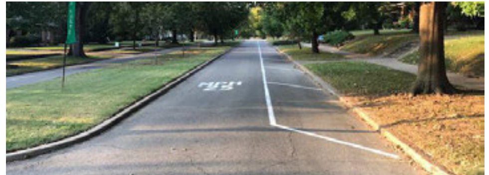
BPAC painted lane markings and the speed limit on an overly-wide street in the Maple Ridge neighborhood in an effort to slow traffic in the area. Photo: BPAC
