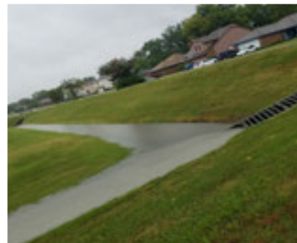
THE NORTH EAST CORNER OF THE DETENTION BASIN
