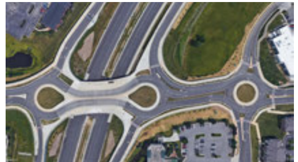
Roundabouts at Highway Intersections, Carmel, IN (Image Source- Google Earth)
