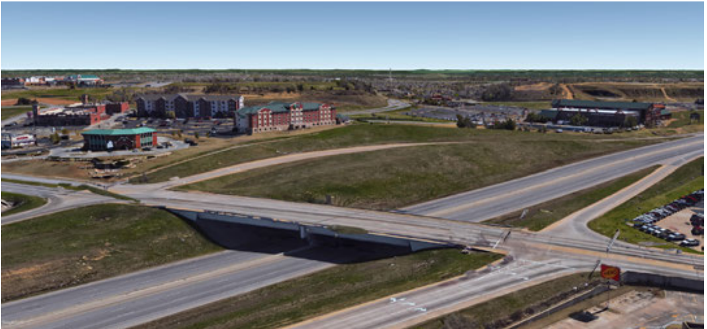
Existing Elm PI- Broken Arrow Expressway Intersection
