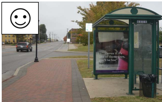
This bus stop is familiar to Tulsans and it provides comfort with shade and seating.
