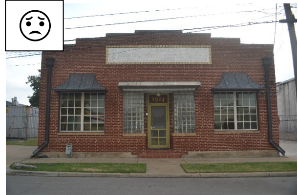
The purpose of this building is not easy to recognize. It is an architectural roofing and sheet metal shop.
