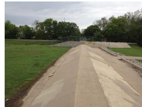
Weir - View West
