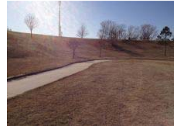
Levee Wall -ViewWest
