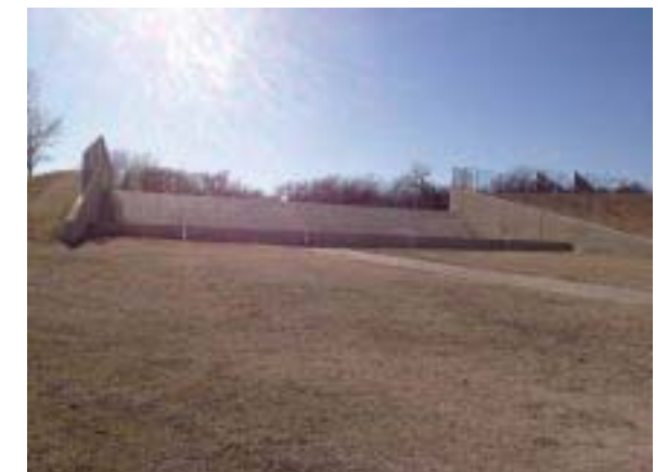
Weir -View West
