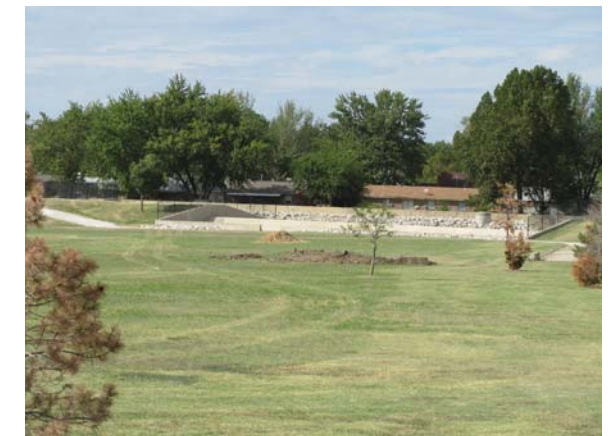
Weir -View Northeast
