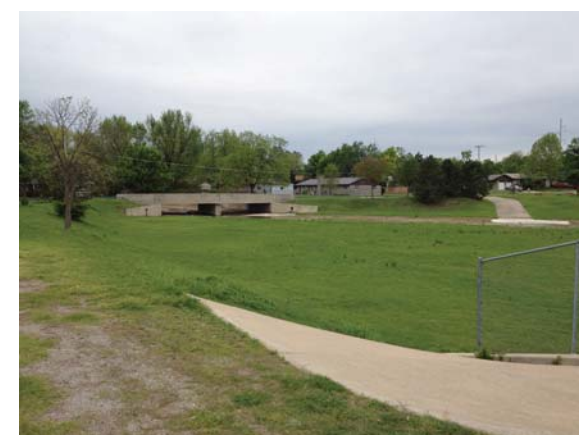
Bridge - View South
