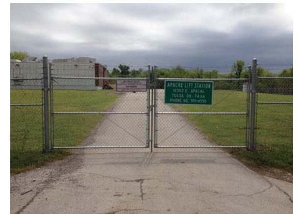
Sewage Pump Station-View South
