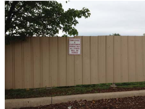
Property Wall - View East
