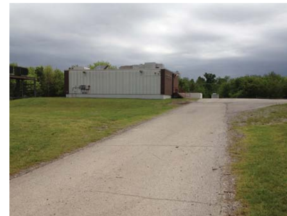
Sewage Pump Station-View South
