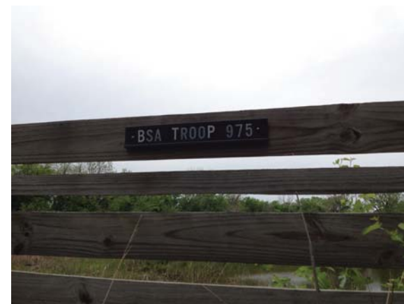
Box Structure-View West
