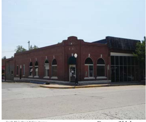
South Main Street & Sims Avenue Depew, Oklahoma Photo Survey Megan Vandecar
