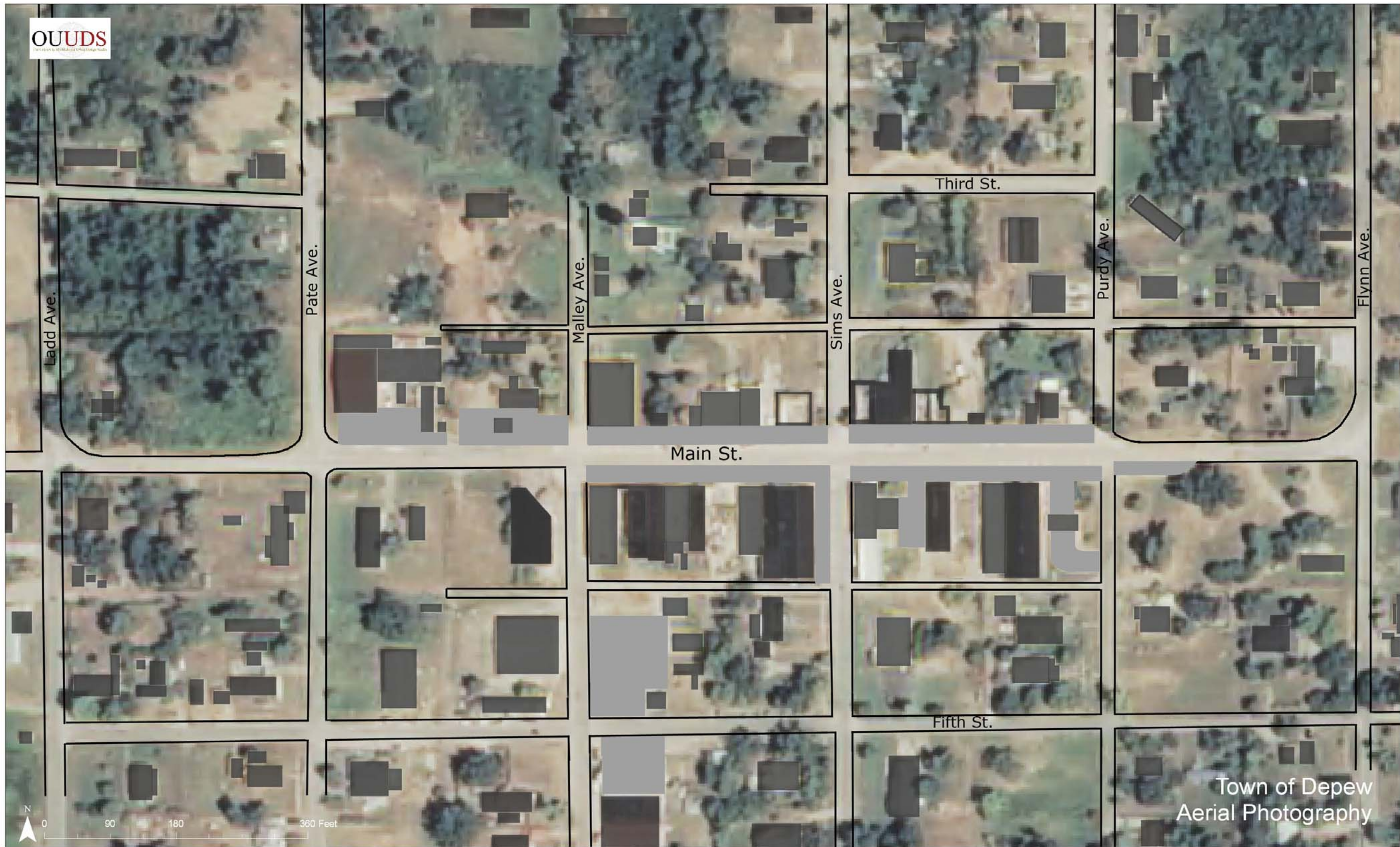
This image clearly shows the corner curves at the ends of Main Street where Route 66 previously traveled through town. Also shown are building footprints and impermeable ground cover. Some of the oldest buildings on Main Street are located between Malley Avenue and Purdy Avenue. Several other historic buildings were lost to fire or tornado many decades ago between Pate Avenue and Malley Avenue.
