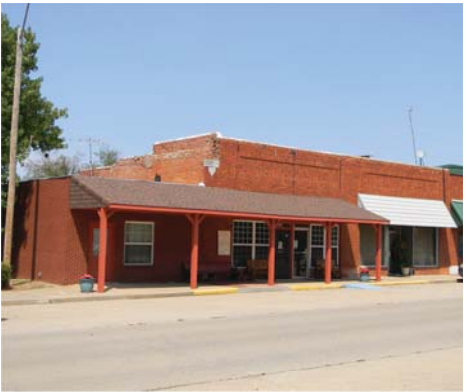
North Main Street between Malley Avenue & Sims Avenue Depew, Oklahoma Photo Survey Megan Vandecar
