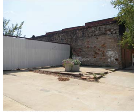
South Main Street between Malley Avenue & Sims Avenue Depew, Oklahoma Photo Survey Megan Vandecar
