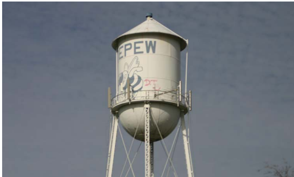
Depew water tower
