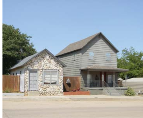
North Main Street & Parady Avenue Depew, Oklahoma Photo Survey Meagan Vandecar OUUDS
