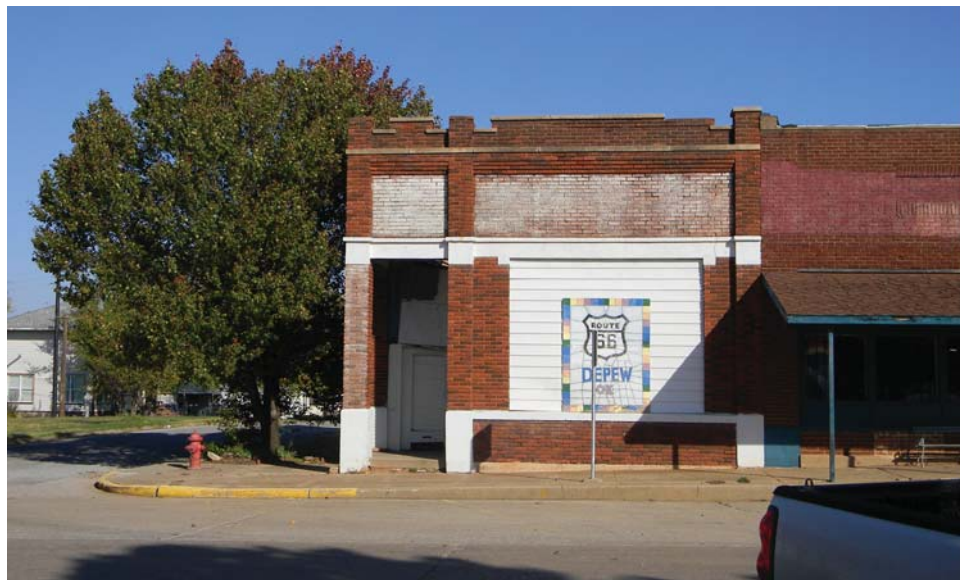
The original First National Bank, now only the facade remains
