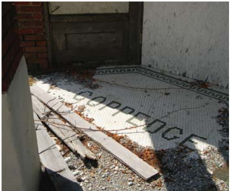
North Main Street & Sims Avenue Depew, Oklahoma Photo Survey Meagan Vandecar OUUDS
