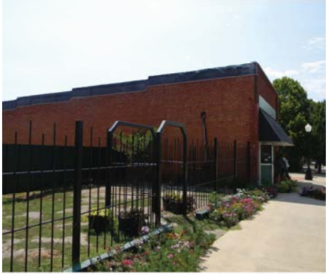
South Main Street & Sims Avenue Depew, Oklahoma Photo Survey Meagan Vandecar OUUDS
