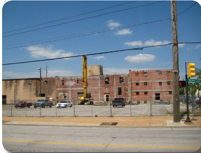
Warehouse in Brady District currently under renovation, Archer and Cincinnati.
