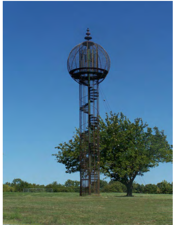
BRUCE GOFF TOWER IN SOONER PARK
