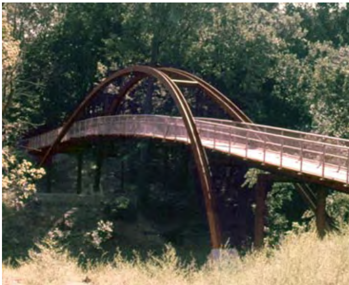
PATHFINDER PARKWAY PEDESTRIAN BRIDGE (IMAGE FROM WWW.BARTLESVILLEPARKS.COM)
