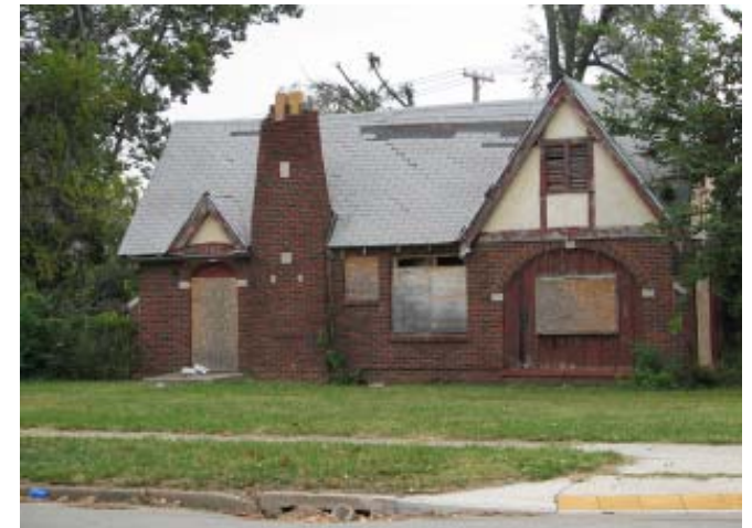
Decaying home in Burroughs neighborhood
