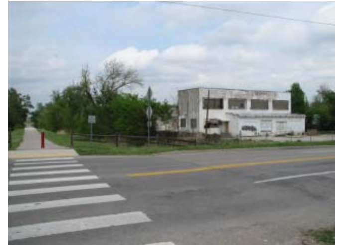
Before: An abandoned brownfield at Apache and the Midland Trail
