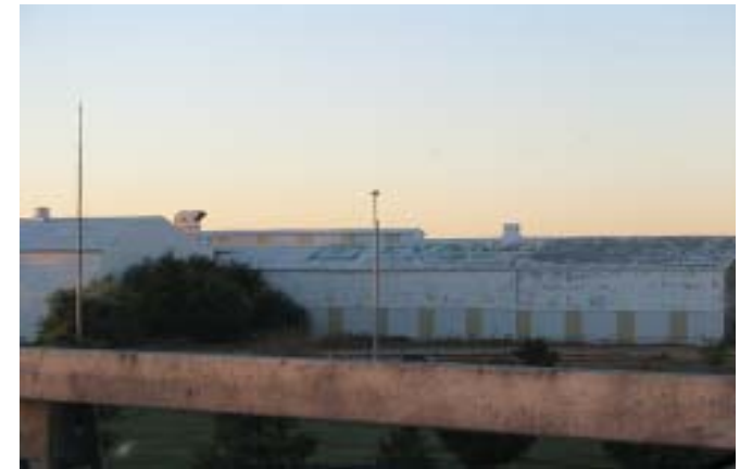
Evans-Fintube site as viewed looking west from U.S. 75
