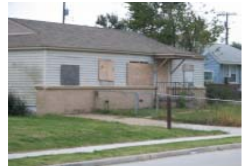
Decaying North Tulsa house
