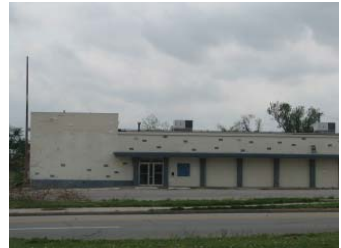
Unutilized greyfield site
