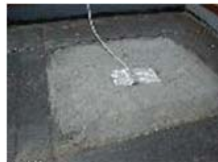
Thermocouple adhered to the roof membrane before adding the drainage layer.
