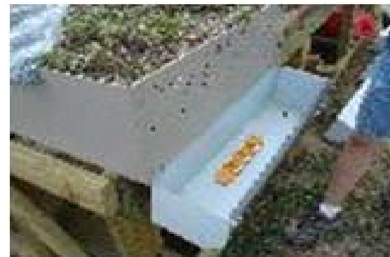
Installing the gutter on a test panel.
