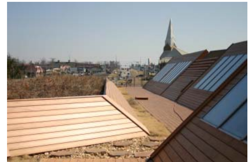
Green roof on the Green Circle Shopping Center facing east.
