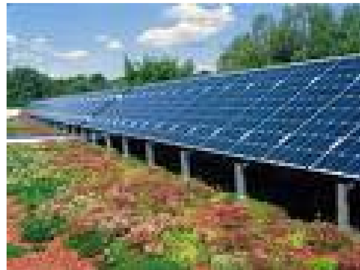
Photovoltaic cells mounted on an extensive green roof. Photo: www.greenroofs.com
