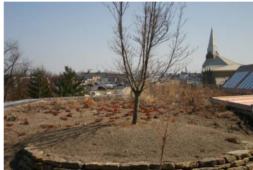
The depth of this tree pit will provide several inches of protection to insect communities that may colonize in the substrate. Photo: Nathan Diekelman
