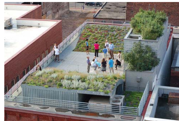
Green roof patio recently constructed on the headquarters of the American Society of Landscape Architects. Photo: www.asla.org
