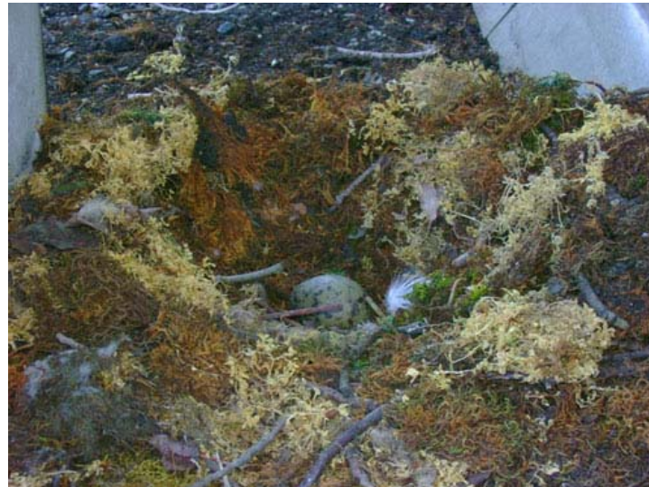
Goose nest on a green roof in Toronto. Photo credit: www.toronto.ca/greenroofs
