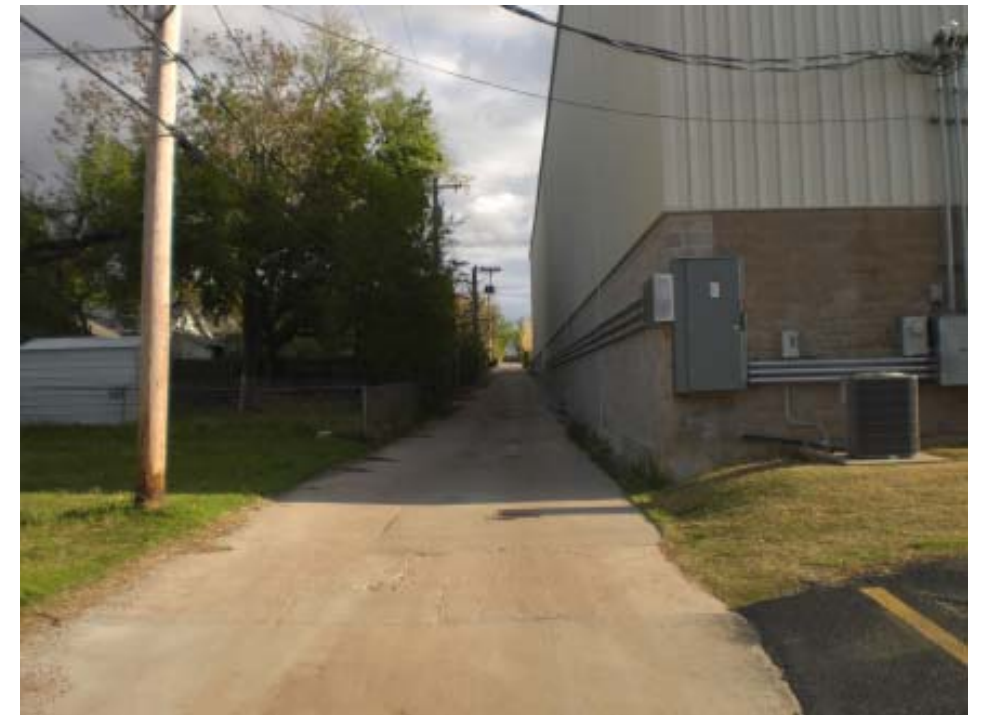
(Above) An alley just off Peoria Avenue is underutilized. By the resident using the alley to park, this is another space to eliminate the potential for criminal activity by having “eyes on the street”.
