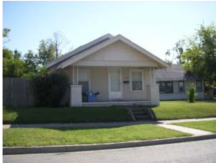
(Above) A typical single-family bungalow on 12th Street between Trenton and Rockford Avenues.
