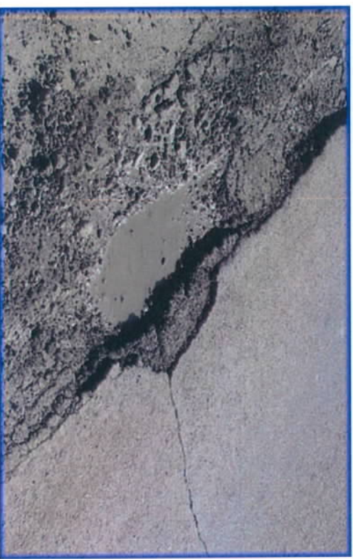
Typical Street condition on Yale Avenue.
