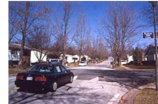
Eugene, OR - This raised crosswalk uses a unique pattern of concrete and brick. Bollards are provided to assist visually-impaired pedestrians detect the beginning of the crosswalk.
