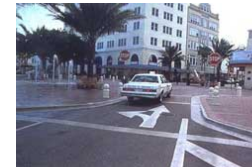
Tallahassee, FL - This raised crosswalk has a profile that more closely resembles a Speed Hump than a Speed Table.
