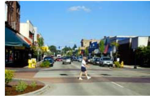
Beaverton, OR - This raised crosswalk uses asphalt and highly-visible paint.
