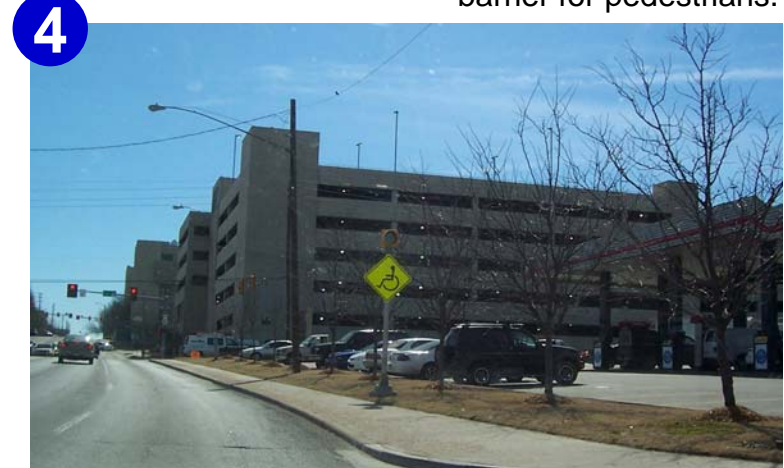
4 Sidewalks close to 11 th St. and Handicap sign.
