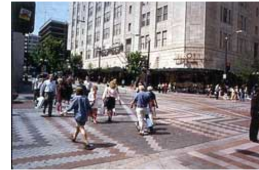
Seattle, WA - This textured pavement covers an entire downtown block and the two endpoint intersections. It is also combined with neckdowns, though they are not pictured.
