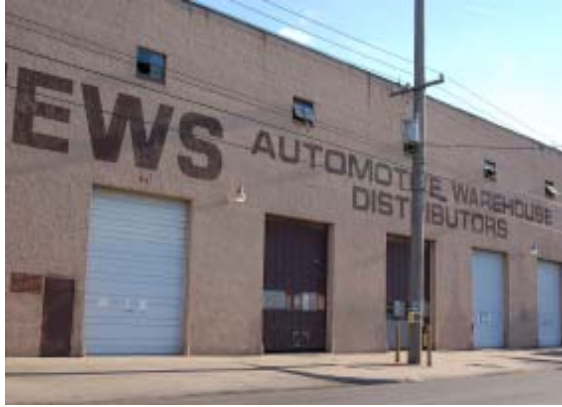
A view of Mathews Warehouse along Brady Street
