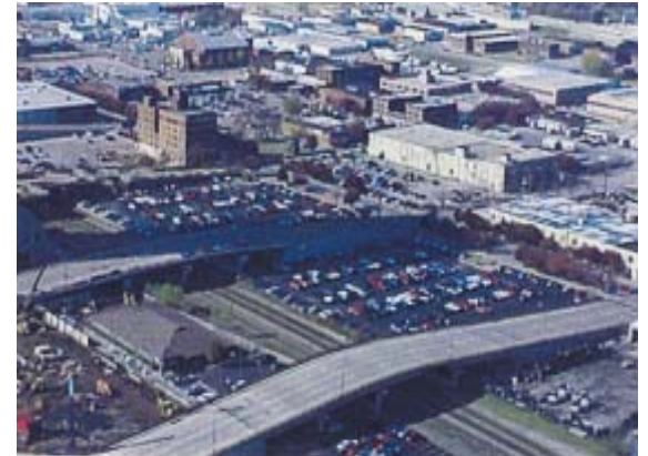
A view west-northwest towards I-244
