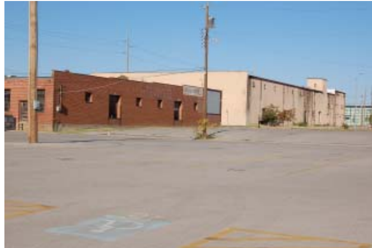
Existing conditions along Brady (between Detroit and Cincinnati).
