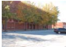
A view of a typical brick building
