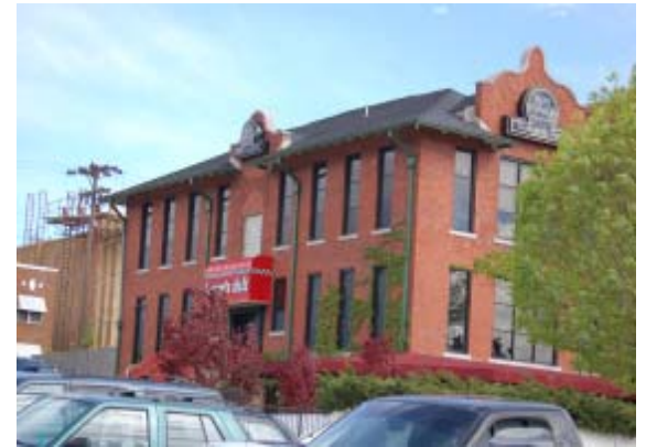
A view of historical building renovated along 15th Street (Cherry Street).
