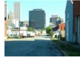
Examples of infrastructure needing repair
