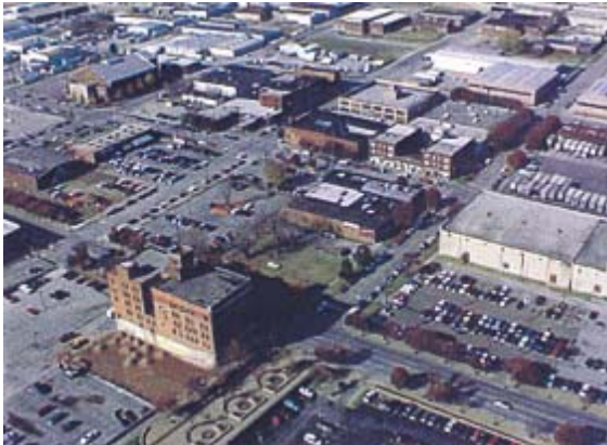
A view northwest
