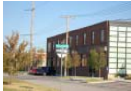
Recently renovated building
