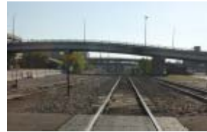
A view west from Boston toward the Main Bridge
