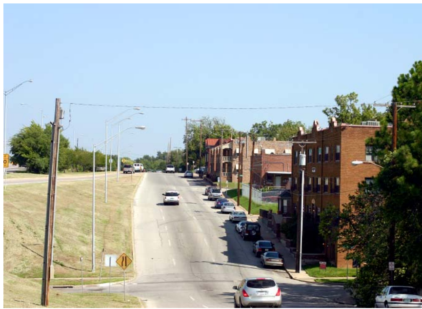
Looking east on the Broken Arrow Expressway service road
