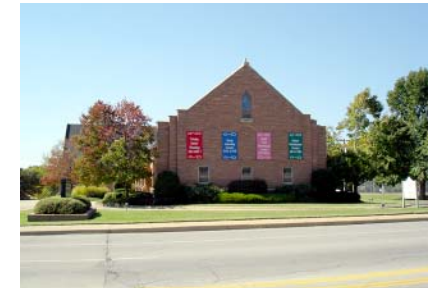
First Lutheran Church, 13th/Utica (west side)
