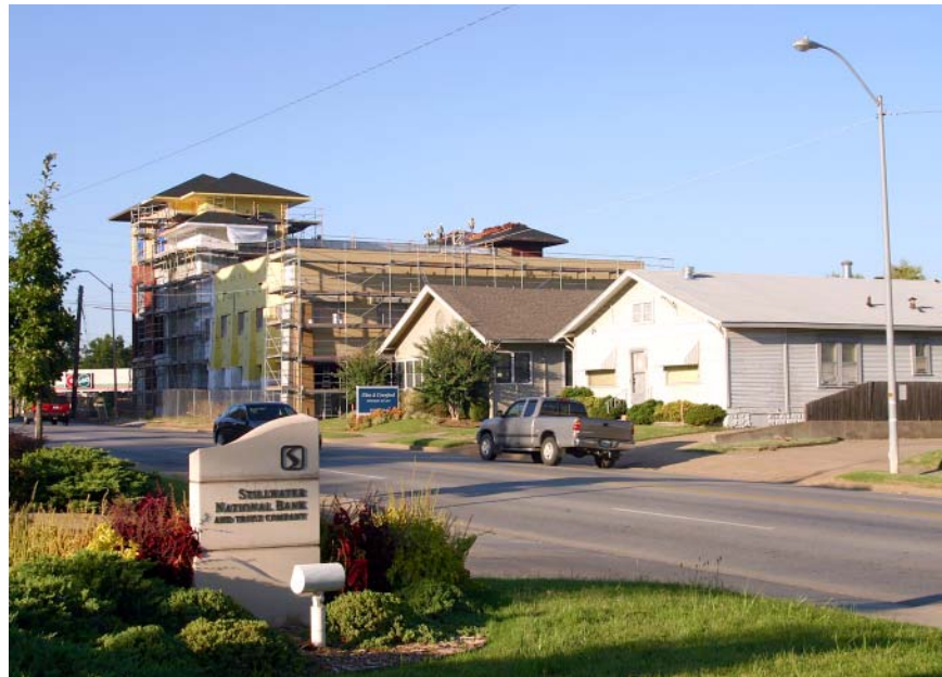
Arvest Bank next to existing structures
