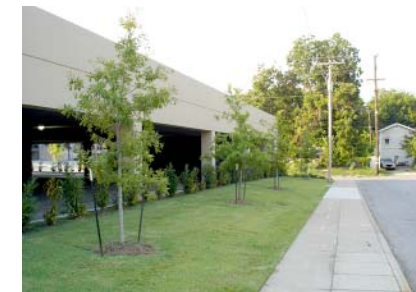
E. side, parking ramp, 12th St. & Wheeling
