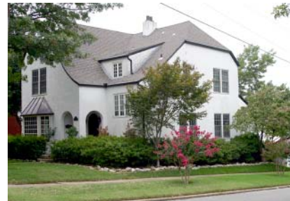
17th and Quaker, SW corner
