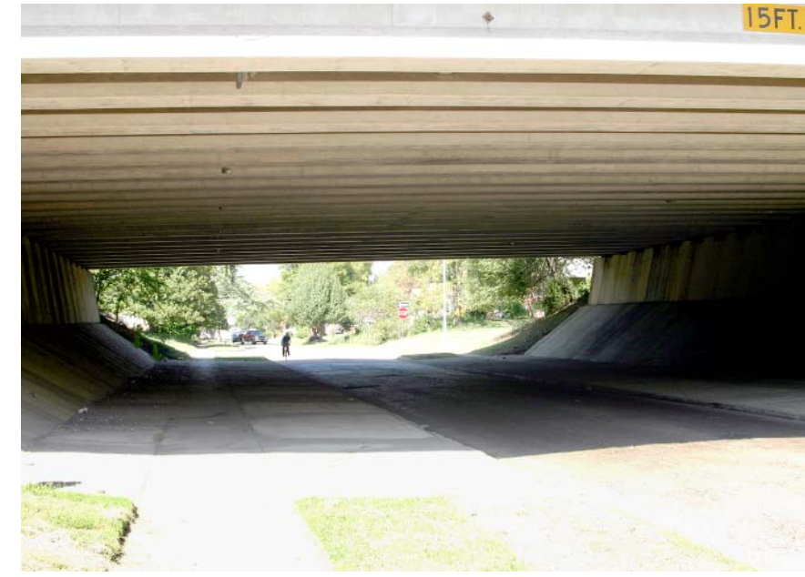
Underpass Broken Arrow Expressway, St. Louis Avenue
