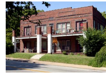
Apartments, NW corner, 13th & St. Louis
