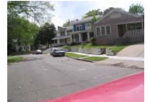
Homes on Elgin. Most of these houses have been condemned or torn down. Photo by Patrick Fox
