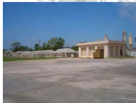
Photo looking North, toward the entrance to the concrete plant.
