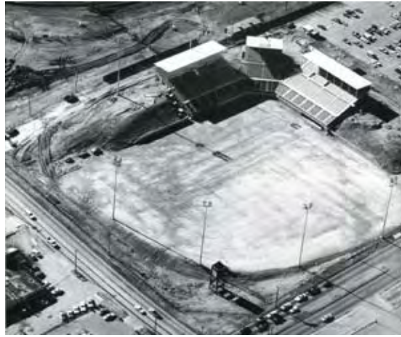
The new baseball stadium under construction in 1980, McCombs pg. 82.
